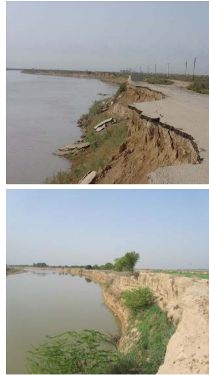
Fig. 3: Karoon river erosion in area of Malihan and Suichi villages (8 and 23 meanders)
