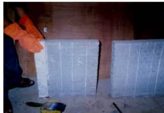
Fig. 1: Wall panels getting ready for GFRP laminations
