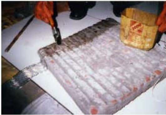
Fig. 2: Polyester resin coating is applied to fix GFRP lamination
