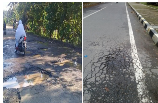
Fig. 1: Expansive soil conditions on the Takalar-Jeneponto highway
