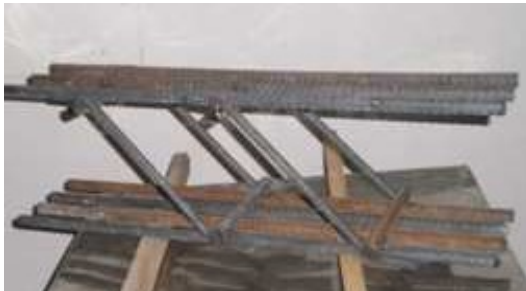
Fig. 2: Typical welded swimmer bars used in beams
