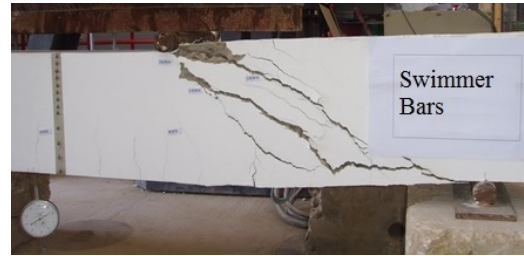
Fig. 13: Typical shear failure
