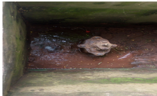
Fig. 6: Leaking control valve at Ikejiani street UNN
