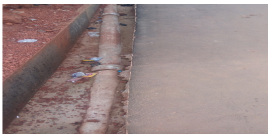
Fig. 2: Drainage line of the newly constructed Sam Onyishi Road. The drainage line was constructed on the main lines to the Odenigwe Reservoir, this could cause pipe bursting during the excavation of the drainage line
