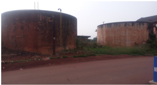
Fig. 1: Abandoned Odenigwe UNN twin reservoir. It has a combined capacity of 1376 m 3 . (Odenigwe, Nsukka)
