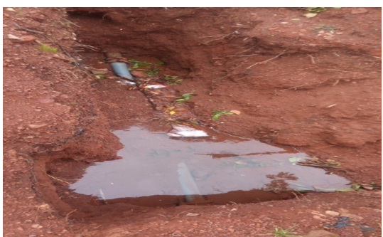
Fig. 3: Leaking pipe at one of the minor lines along Ikejiani Avenue, UNN
