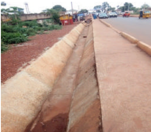
Fig. 6: Well-constructed drainage system in Enugu Road
