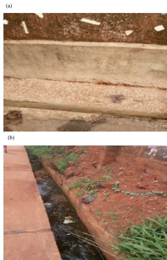
Fig. 24: a) Stone pitching method at University Market-Road and b) Un-stone pitched soil mass in Odenigbo Road
