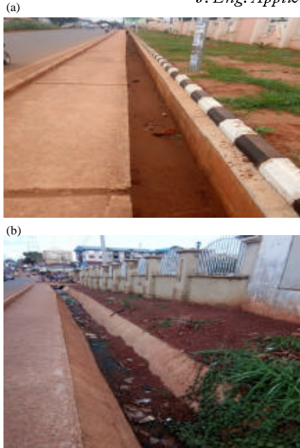
Fig. 25: a) Cementing method with kerb in Odenigbo Road and b) Un-cemented soil mass at Enugu Road
