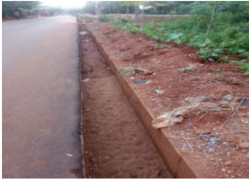
Fig. 16: Farm land along Odenigwe Road that dissipates fine particles into the drainage system during rain
