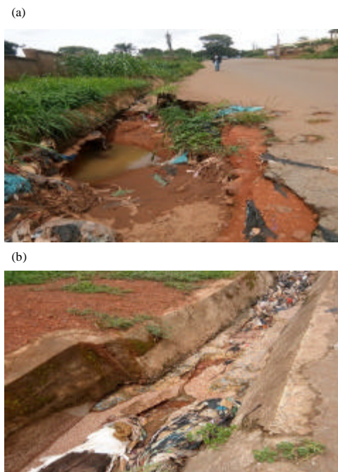
Fig. 22: a, b) Roads with temporary waste site, very poor waste managements and poor drainage condition, e.g., University market-Road
