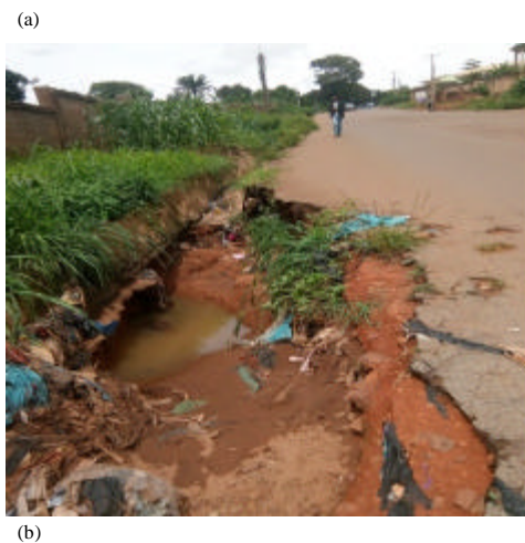
Fig. 8: Section of poorly constructed drainage system in Odenigwe-Road
