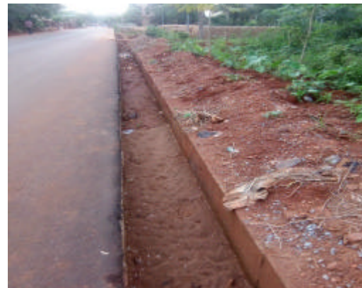
Fig. 15: Drainage section where latitudinal siltation should be prevented in Orba-Road
