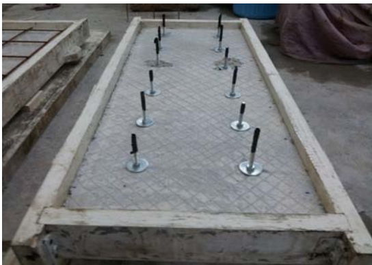
Fig. 3: Shear connector's distribution
