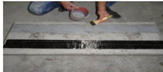
Fig. 5: Placement of CFRP sheets
