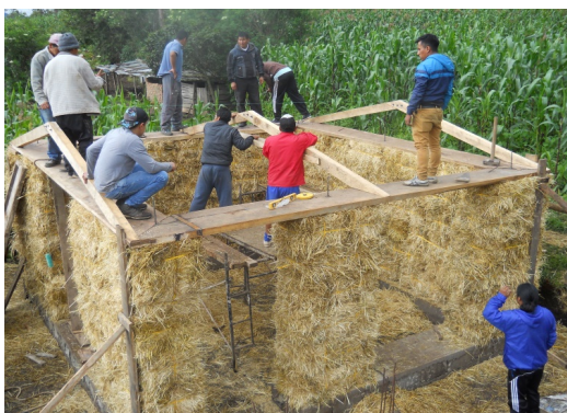
Fig. 13: Perimeter beams and wooden trusses
