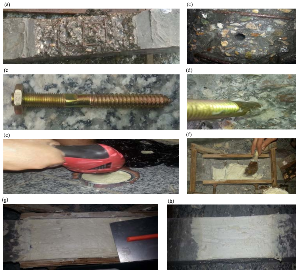
Fig. 4: Repairing with polyester glue line: a) Clean the damaged zone; b) Hole of shear connector; c) Shear connector; d) Fixed shear connector; e) Mixing polyester glue line; f) Pervading polyester glue line; g) Adjustment polyester glue line and h) Repaired damaged zone
