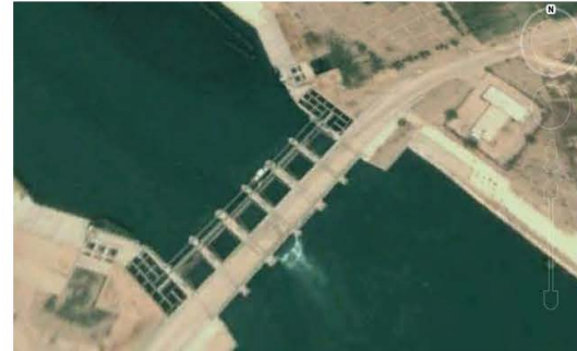
Fig. 2: The flood control structure under study
