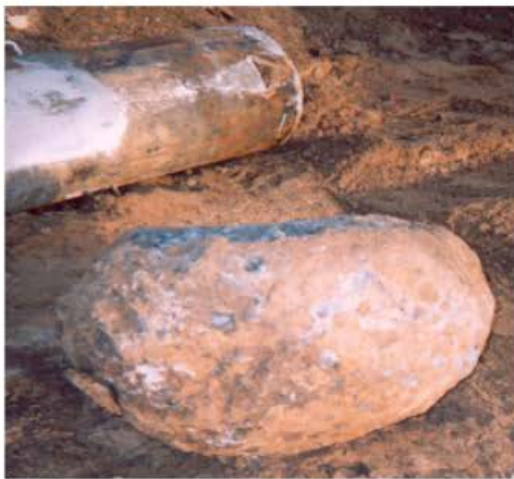
Fig. 12: The cases-punch with butt plugged end and excavated rammed pedestal under the pile toe
