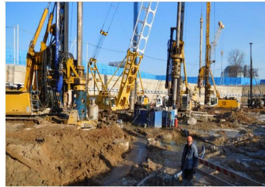
Fig. 5: Drilling of wells by drilling rigs of the firms "Bauer" and "Cassagrande" under the protection of casing pipes with scooping out of the ground by bailers and refilling of water into the casing
