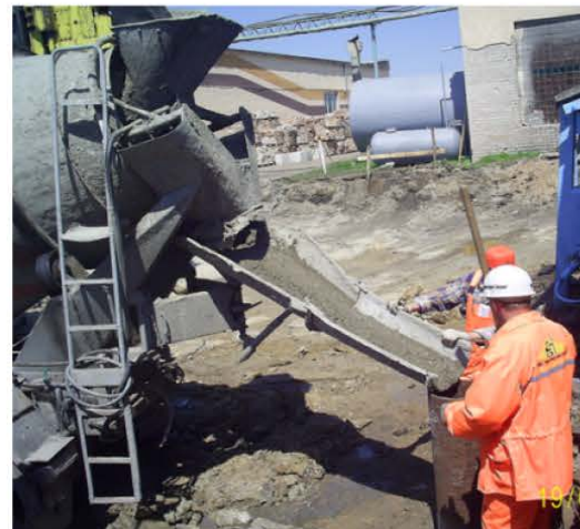
Fig. 10: Concreting of the casing shaft by mixer
