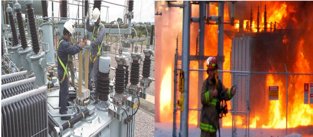
Fig. 1: Transformers and machines in Morupule Power Station (Anonymous, 2017)
