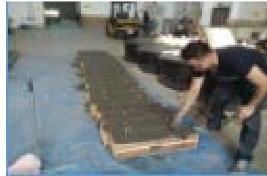
Fig. 1: Concrete casting of RC beam
