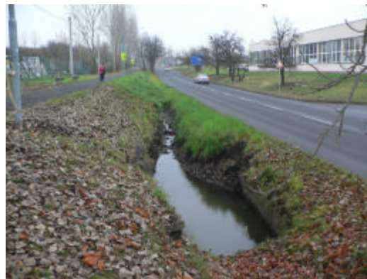
Fig. 3: Photo documentation - general view of the LRSCD in the direction of the roundabout at the connection of Jirasek-Lomska-S.K. Neumann streets; the catch-drain is not maintained. With proper function of the pipe underpass, the water should be transferred to the opposite side of the local road and further through the concrete DN 200 relief sewer into the Divoky potok stream; however, this important concentration and transfer object is in a poor state; the inlet to the pipe underpass and to the following relief sewer is not secured against inlet of sediments which in connection with absence of operational maintenance had a harmful influence on the permeability of the pipe underpass and to subsequent relief sewers
