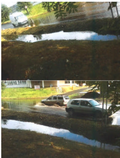
Fig. 1: Photo documentation-the photos showing the emergency state, common danger state at the Kaufland shopping centre caused by insufficient of the Local Road Space Catch Drain (LRSCD) at Jirasek and insufficient function of the follow-up concentration and transfer object of the (LRSCD) and the relief sewer
