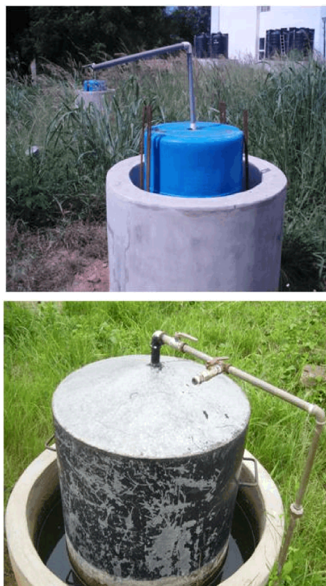
Fig. 6: (a) A Broken down twin floating-drum plant at GIMPA; (b) Abandoned floating-drum plant at Tepa slaughterhouse
