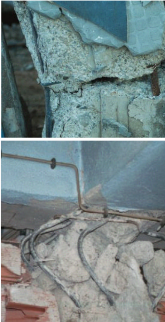
Fig. 6: Insufficient material and detail in a column
