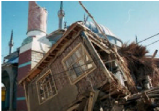
Fig. 9: Highly damaged non-engineered structure
