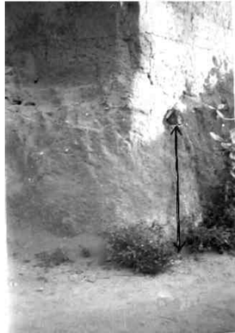
Fig. 2: Foundation of a mudhouse exposed by 1.2 m (shown with arrow) by sheet erosion and street floods over duricrust concretions within the built-up areas (site A in Fig. 1)
